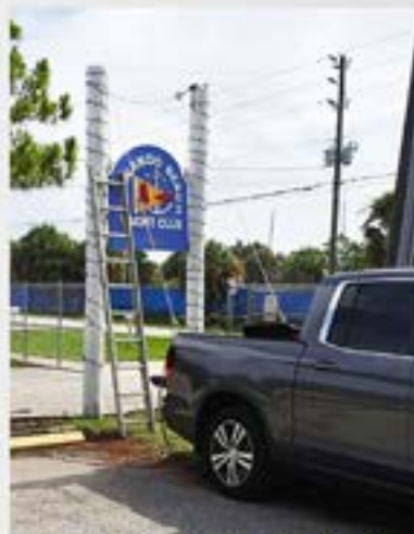
Hoisting the sign by pickup truck
