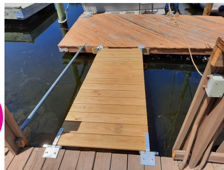
All HBYC dock ramp corroded hinges (left) were replaced and a new dock ramp replaced the old south end dock ramp (right).
