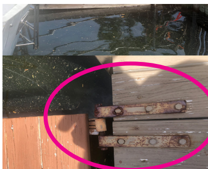
All HBYC dock ramp corroded hinges (left) were replaced and a new dock ramp replaced the old south end dock ramp (right).
